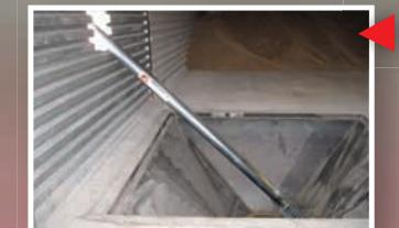
A reception pit built into the floor inside the grain store allows trailers to be tipped quickly but would require a large capacity auger to feed straight into a Dryer without a pre store bin
