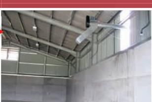
A horizontal discharge auger discharges through the cladding and over the grain walling of the dry grain shed to finish the process
