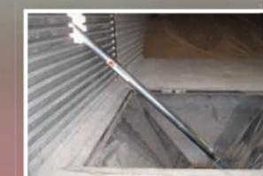
A reception pit built into the floor inside the grain store allows trailers to be tipped quickly but would require a large capacity auger to feed straight into a Dryer without a pre store bin
